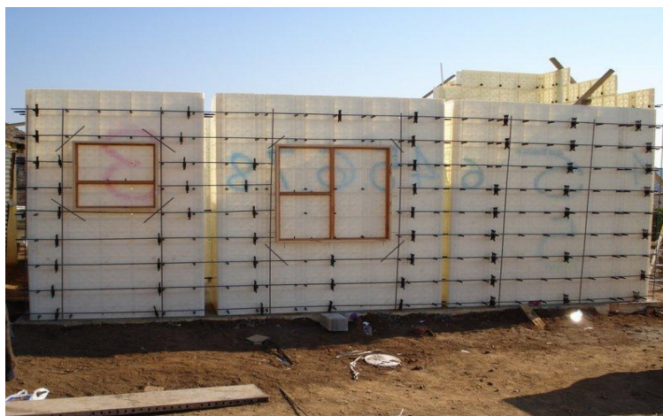
Fig 1.3 plastic formwork
