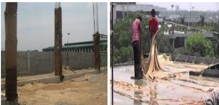
Fig 3.3 Covering concrete surfaces
