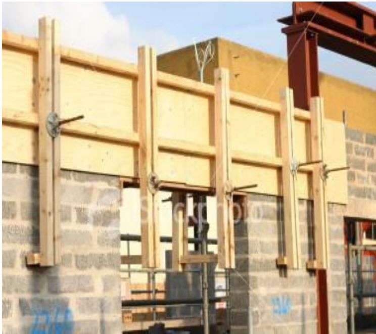
Fig 1.1.1 timber formwork
